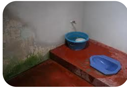
Toilet inside after
