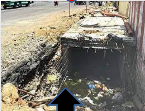
The So Called Storm Water Drainage
