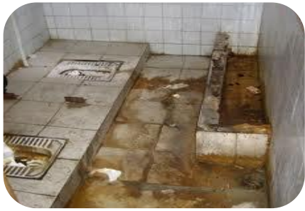
Toilet Inside before
