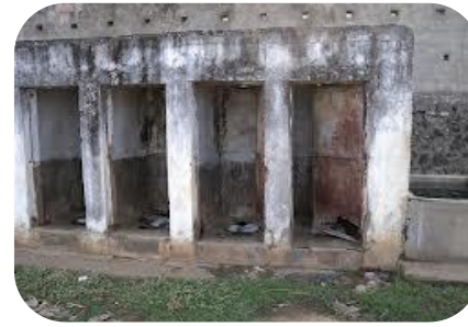
Public Toilet Before
