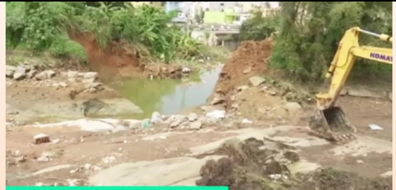
Hulimavu Lake bund breach, several houses flooded in Bengaluru
