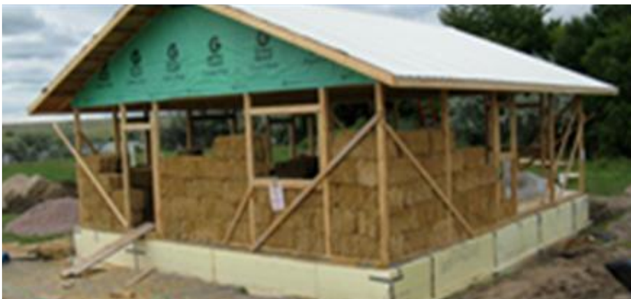
Straw Bale House Under Construction
