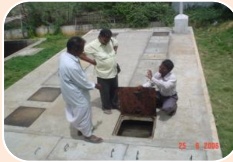
SoLiWaM © Source Liquid Waste Management Toilet Credit Dewats
