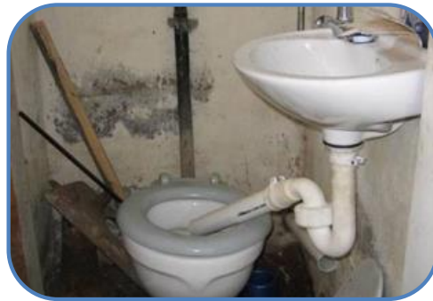
Wash Basin Water waste water flushes toilet
