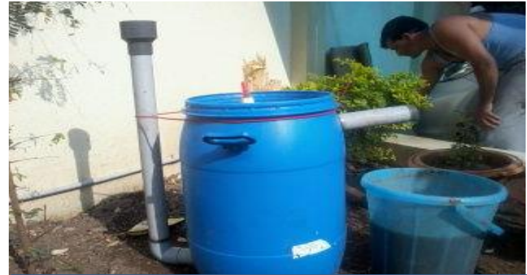
SoGaWaM Source Gas Waste Management
