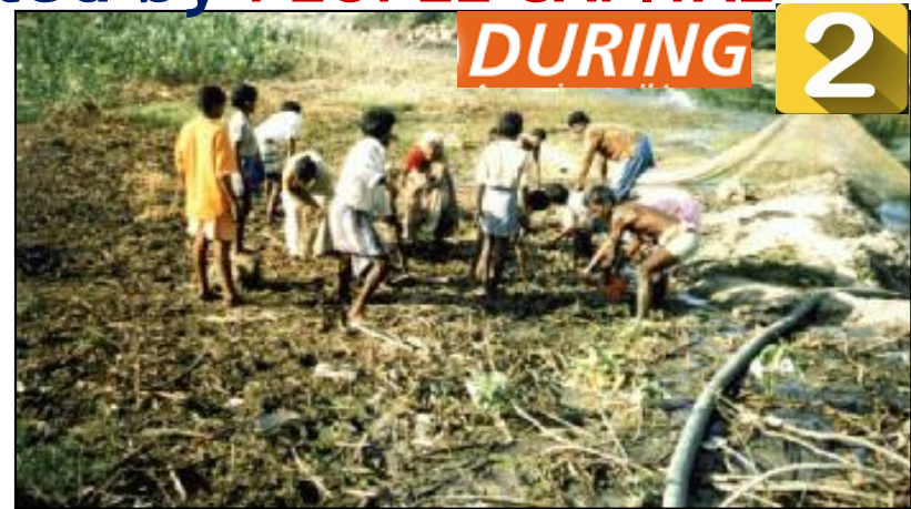
Dewatering & desilting the
