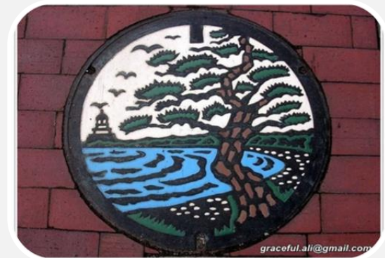
6. Drainage Manhole with an artistic LID
