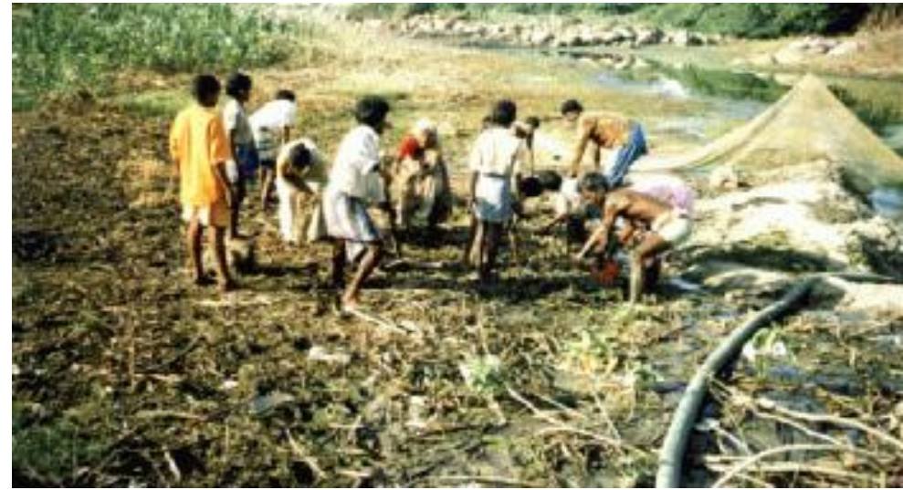
Dewatering & desilting the pond
