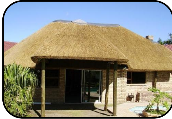
WATER REED ROOF
