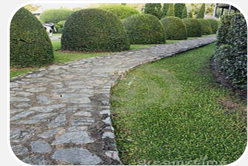
9. Well paved pedestrian path
