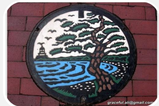
6. Drainage Manhole with an artistic LID
