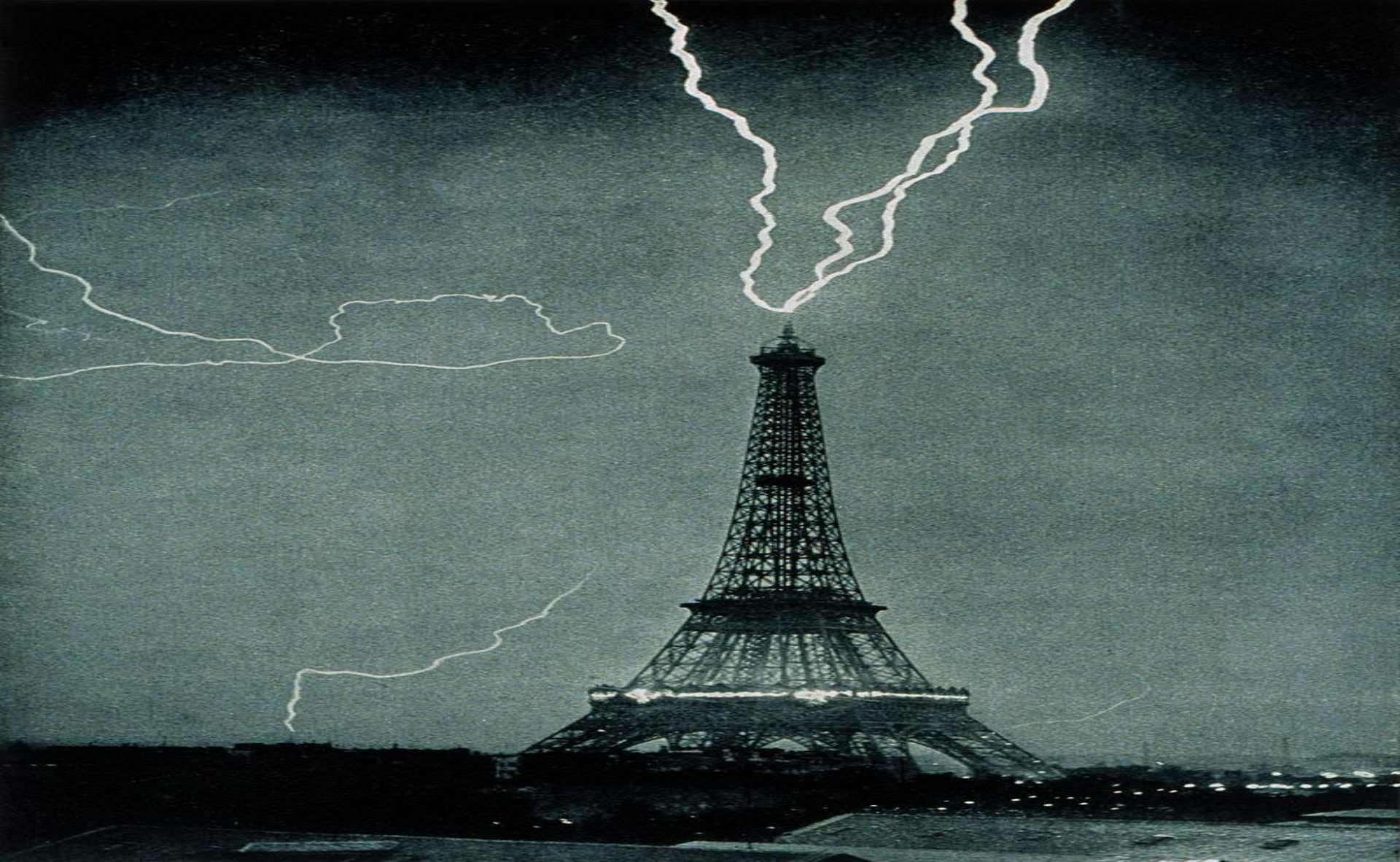
The Eiffel Tower as a colossal lightning conductor. Photograph taken 1902-06-03 21:02
