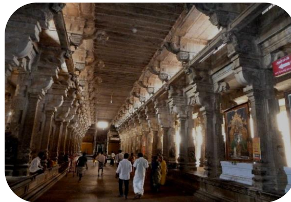
BRICK , MORTAR & GRANITE ROOF
