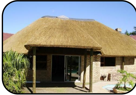
WATER REED ROOF
