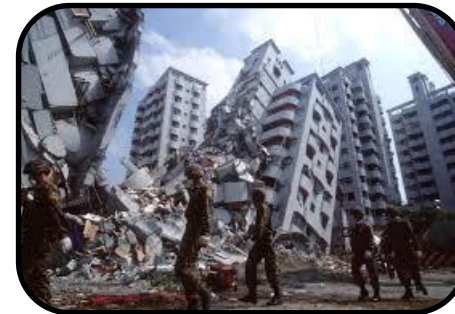
Earthquake due to increased water weight
